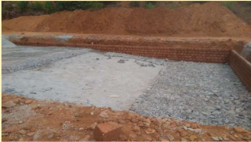
Construction of New Swimming Pool
